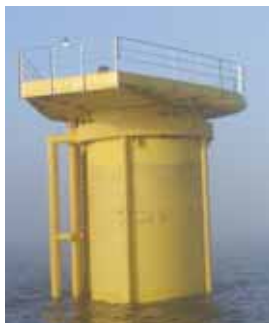
Foundations: MT Hojgaard
