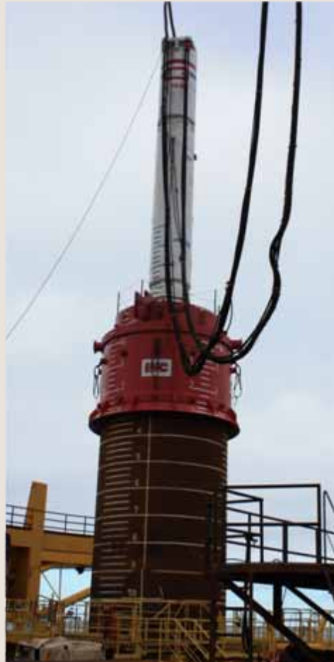
S-1200 Hydrohammer driving 5.100mm piles at Greater Gabbard.
